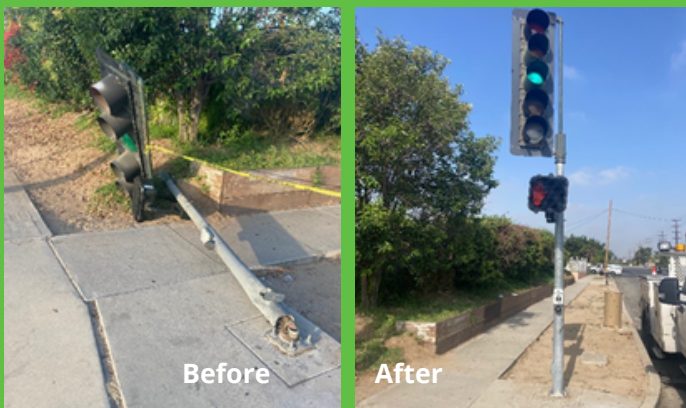
Repaired Traffic Pole at the Intersection of Mill and Eucalyptus (Ward 6)
